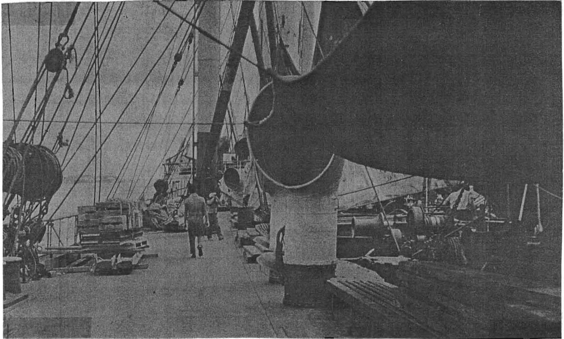
Rain tents were also being rigged . . .
